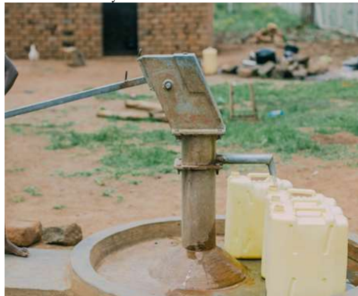
Figure 6: Manually drawn borehole for a community
