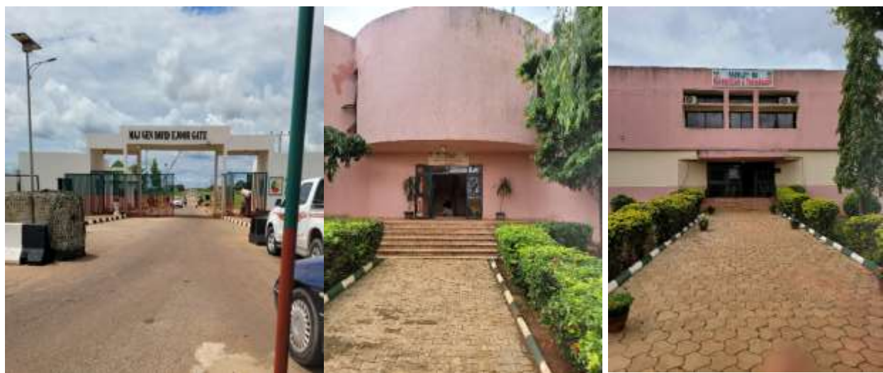
Plate 2: Showing the entrance gate and some faculty buildings at the Nigerian Defense Academy (NDA) with no Handwashing Point (s)/station(s)
